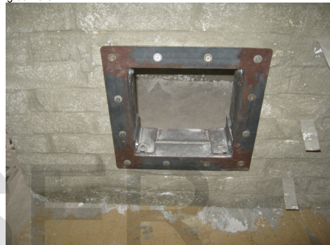
Figure (12) Details of the used rehabilitation technique using steel angle 3x50 mm around opening at both sides welded with steel angle inside opening corners.
