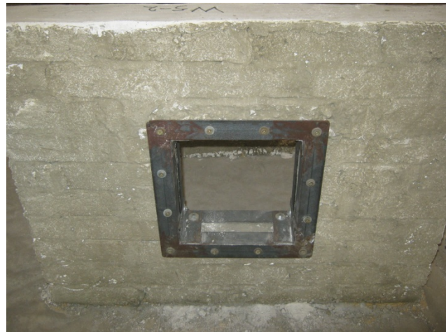
Figure (11) Details of the used rehabilitation technique using steel angle 3x40 mm around opening at both sides welded with steel angle inside opening corners.
